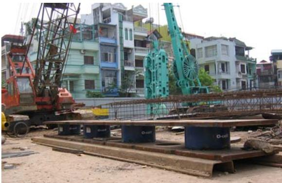
Figure 9.- Bearing plates being assembled to carry the O-cells for the 7 m long barrette
