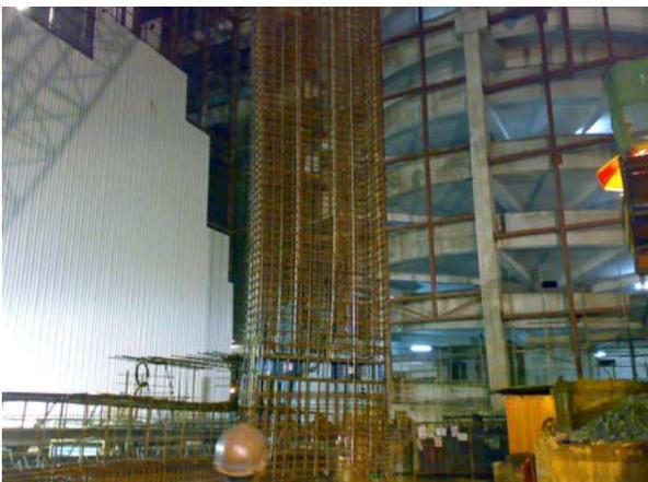
Figure 15.- Installation of the twin 660mm O-cells within the working barrette.
