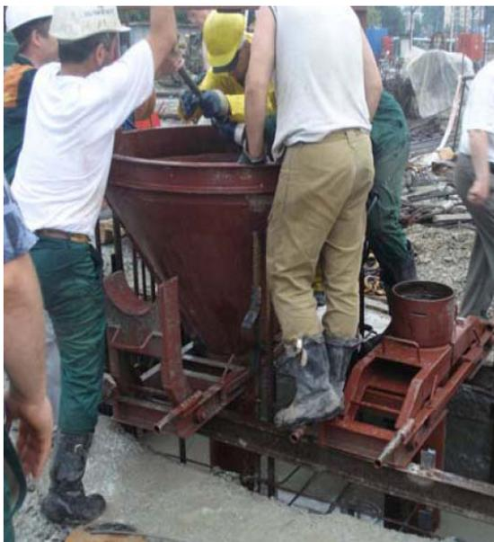
Figure 7.-placement of two tremie pipes for concreting.
