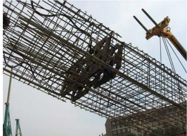
Figure 12.- The O-cell Assembly installed within the barrette reinforcement
