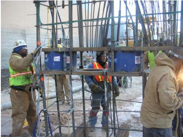
Figure 14.- Cut-outs and funnel arrangements made to allow the use of two tremie pipes during concreting.
