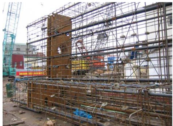
Figure 8.- O-cell bearing plates in position in the barrette cage.
