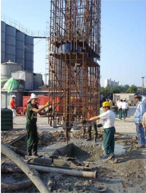
Figure 6.-Installation of barrette cage in the panel.
