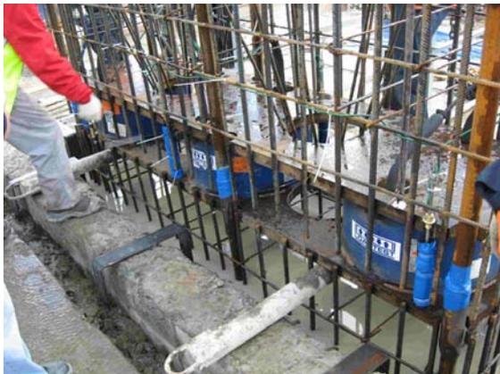
Figure 3. -O-cell assembly installed safely within the barrette steelwork during construction.
